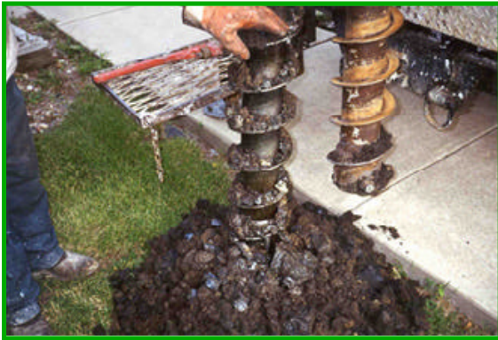
Figure 4. Drilling for the installation of an extraction well.
