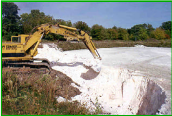
Figure 3. Excavation of lime sludge lagoon.
