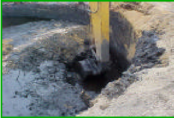
Figure 2c. Excavation of contaminated soil.
