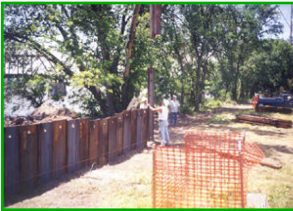
Figure 1. Sheetpile wall installation.
