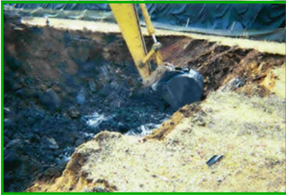
Figure 2a. Excavation of contaminated soil.
