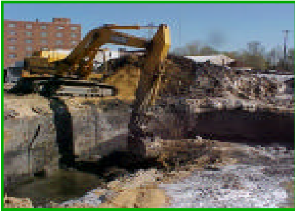
Figure 2b. Excavation of contaminated soil.
