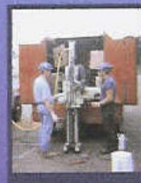
Direct-push injection of slurry.
