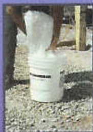
ORC powder is mixed with water to form a slurry.
