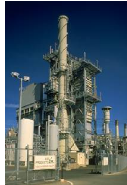
Hydrogen plant in Tosco Corp's Avon refinery 1
