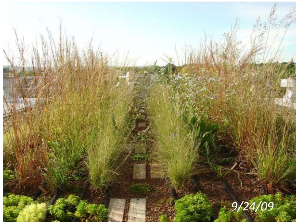
Upper breezeway roof – 300 sq ft; can hold ~64 lbs/sq ft
