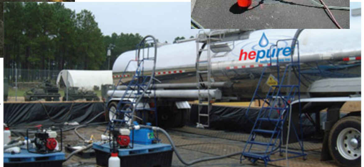
Oxidant Delivery via Pumping
