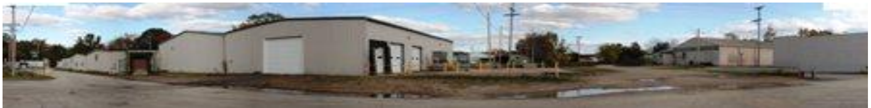
Abandoned industrial buildings in Paw Paw, Michigan which have been impacted by hazardous substances
