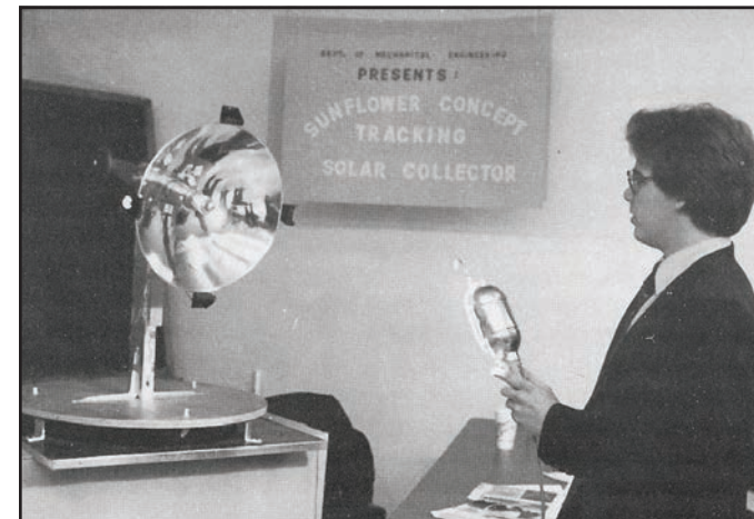
A solar tracking device built by ME students was a winner in the Best Display award category of Open House. The device consisted of a solar collector that moves with the light source.
