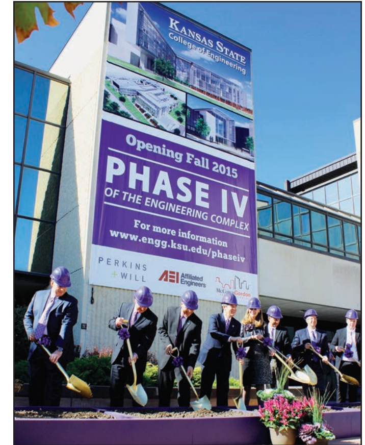
Shovels hit the dirt at ceremonial groundbreaking activities for Phase IV of the engineering complex expansion.
