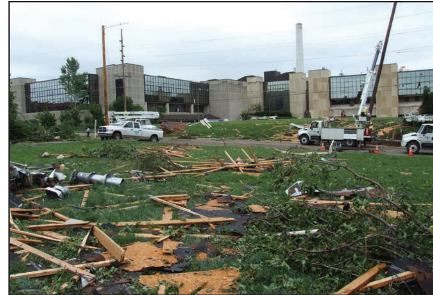
Damage was wide spread from the June 11 tornado outside of the engineering complex.
