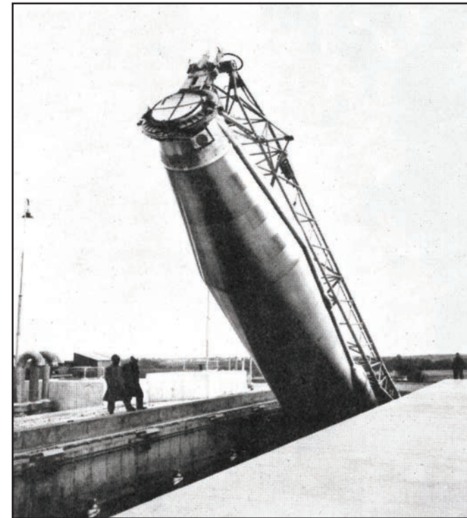
Atlas, America's first operational intercontinental ballistic missile, rises from its pod as the top of the shelter rolls back. Engineers at K-State are converting three area missile silos and associated equipment into tools for teaching and research.
