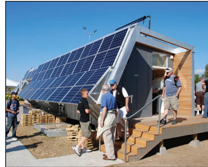
K-State's entry is on display at the 2007 Solar Decathlon on the National Mall in Washington, D.C.
