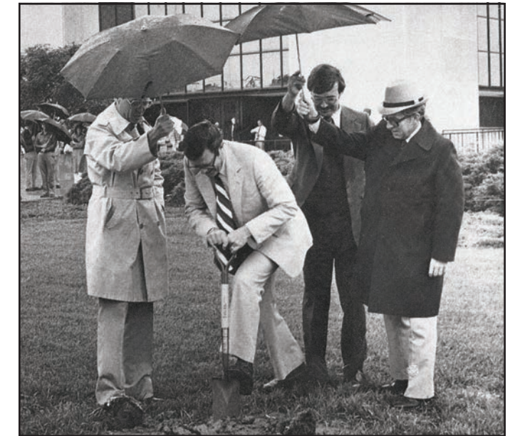
Dean Donald Rathbone turns the first shovelful of earth marking Durland Hall, Phase II ready for construction.
