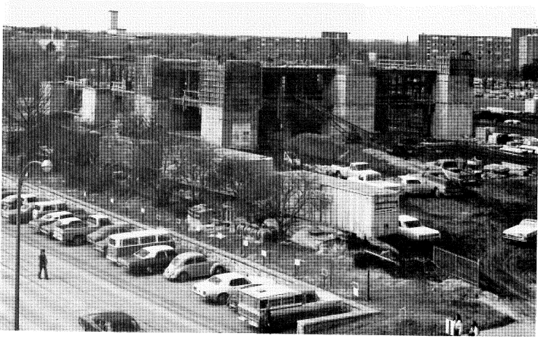
Construction of Durland Hall, Phase I was completed in 1976.
