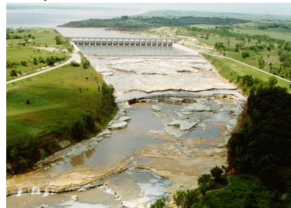
Tuttle Creek Spillway after flood and predicted erosion using WinDAM software
